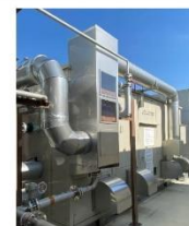
FJ2 is equipped with production lines and an HVAC system that use natural refrigerants, not HHCs (photo: refrigeration system that uses natural refrigerant)
